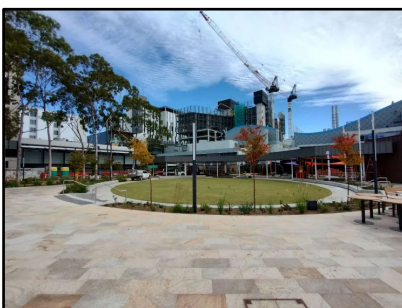
Construction underway for 'KidsPark'
